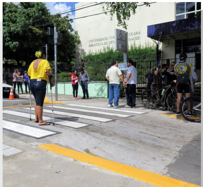
FIGURE 42: RAISED PEDESTRIAN CROSSING IMPLEMENTED AS PART OF THE SUPPORT FOR PEDESTRIANS CIRCULATION PROGRAM
