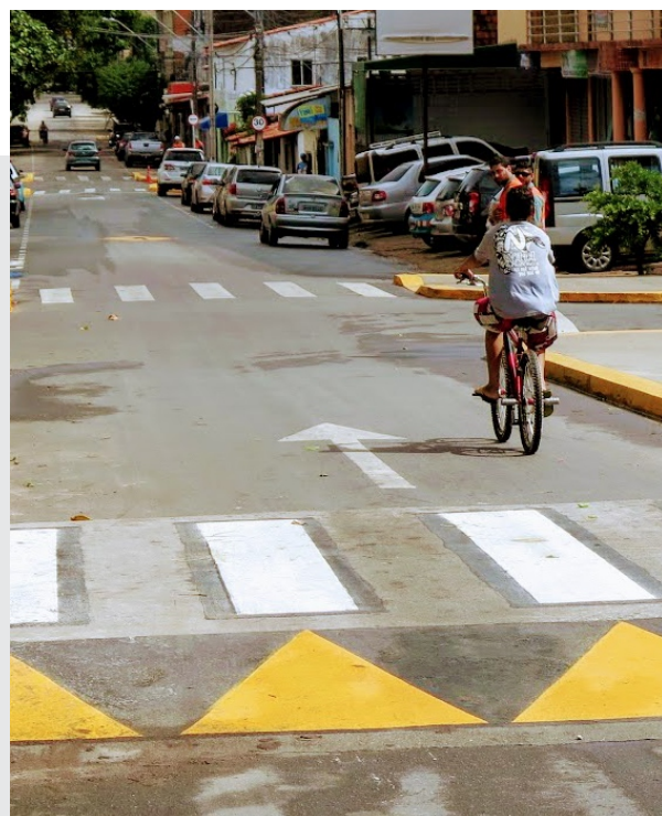
FIGURE 40: RAISED CROSSING, MICRO-ACCESSIBILITY AT SLOW-SPEED ZONE
